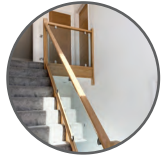
Household Stair Renovations
