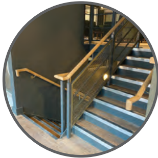
Staircase & Bespoke Fabrications
