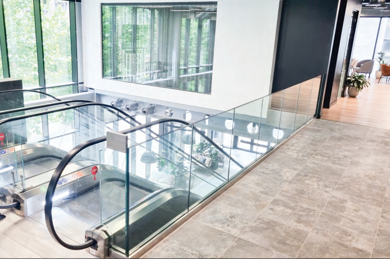
Circle Square 2 Manchester - Stainless Steel Grab Rail With Frameless Glass Balustrade To Upper Level
