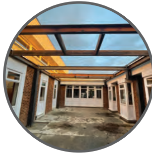
Secondary Steelwork
