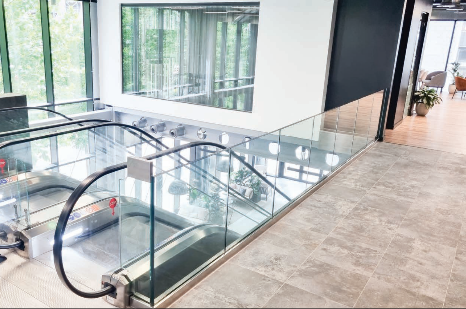
Circle Square 2 Manchester - Stainless Steel Grab Rail With Frameless Glass Balustrade To Upper Level
